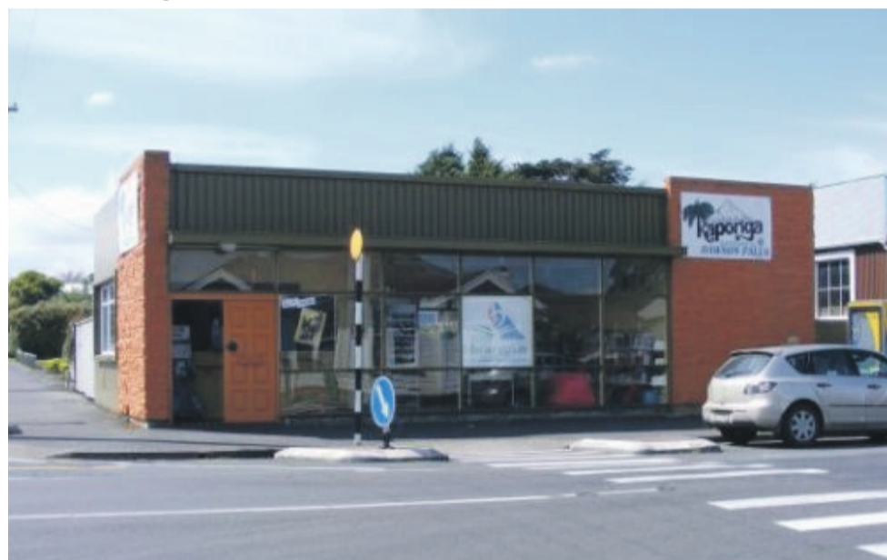
The Kaponga Library due to be earthquake strengthened.
