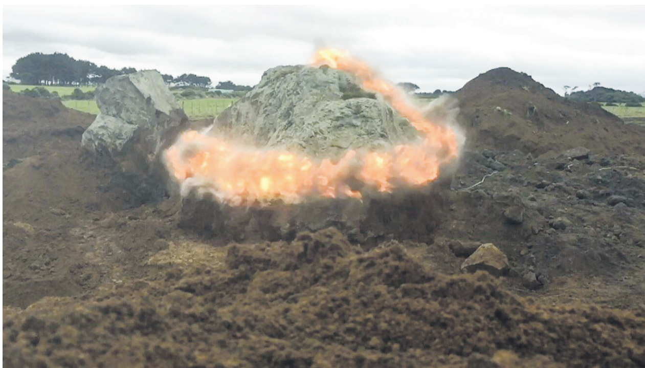
The cortex exploding milliseconds before the rock explodes.
