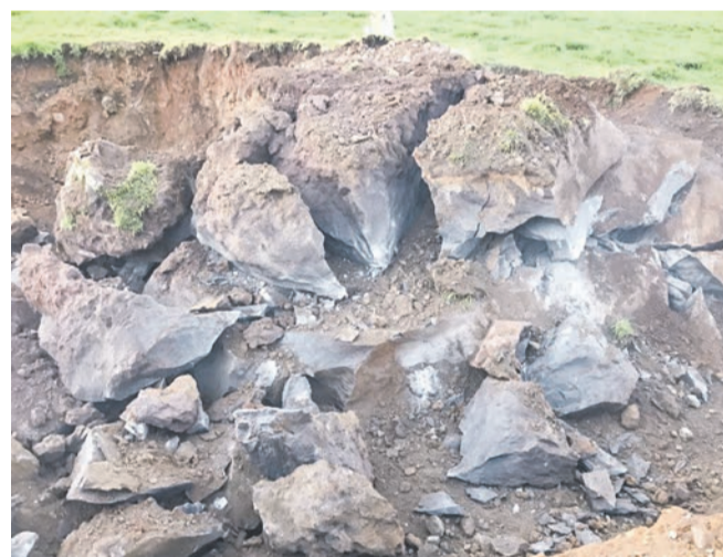
The successful explosion of a ten plug explosion of an estimated 70 tonne boulder blocking a farm track in Wataroa Road.
